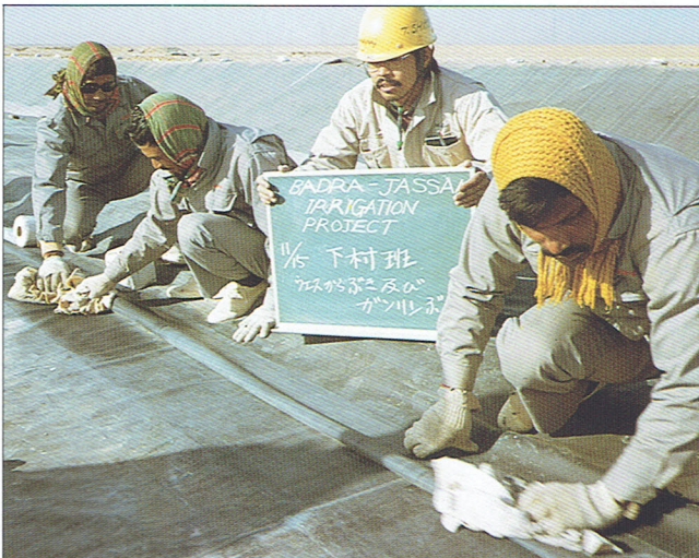
MIZU SHEET is cleaned, RTV-JOINT TAPE is applied to make the splice.
