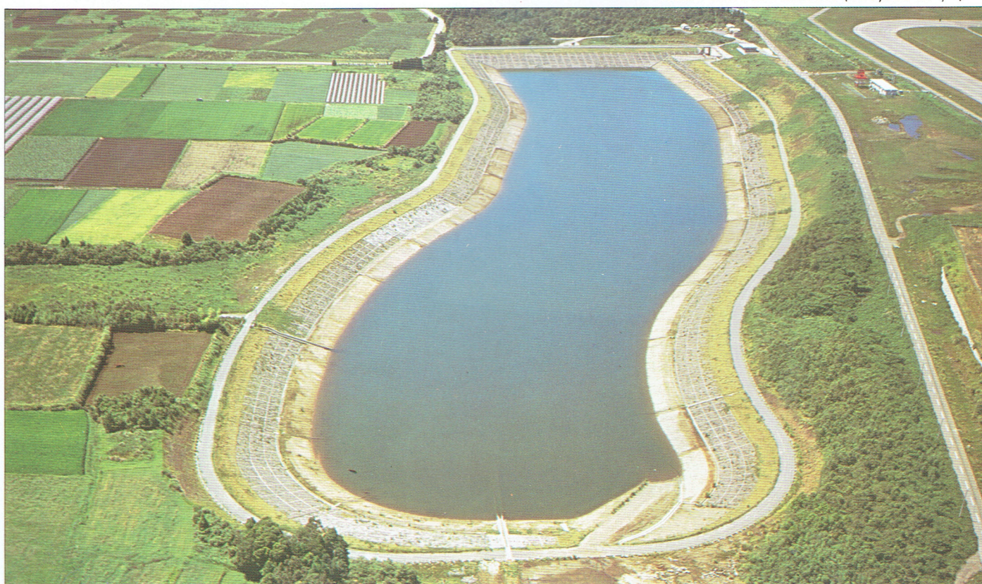
Water Control Facilities (120,000 m 2 ) ▼
