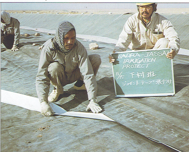
Removing the release paper of RTV-JOINT TAPE
