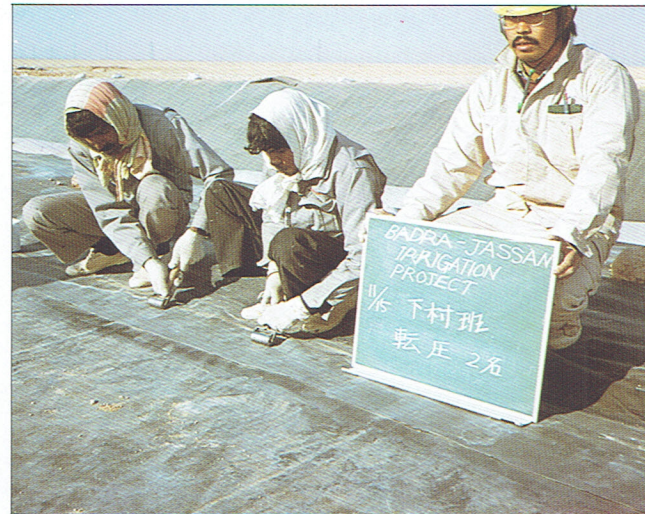
Press down with hand roller
