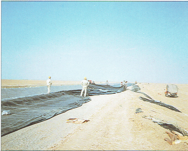
Crew progressively unfolds liner of MIZU SHEET and pulls it up embankmen
